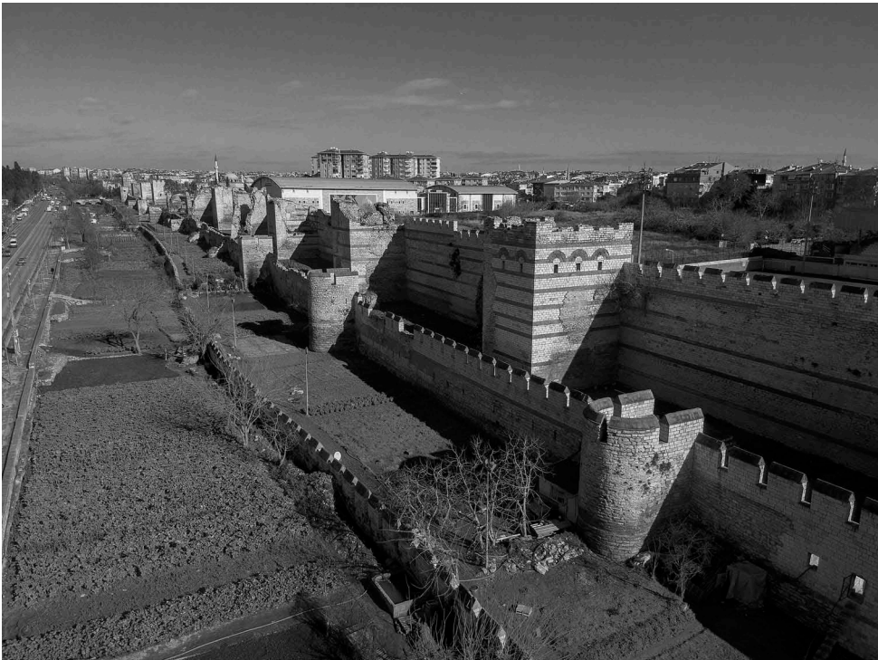
Figure 2.2 The Land Walls of Constantinople, showing their three-tier construction. The site of the moat is now filled with vegetable gardens
